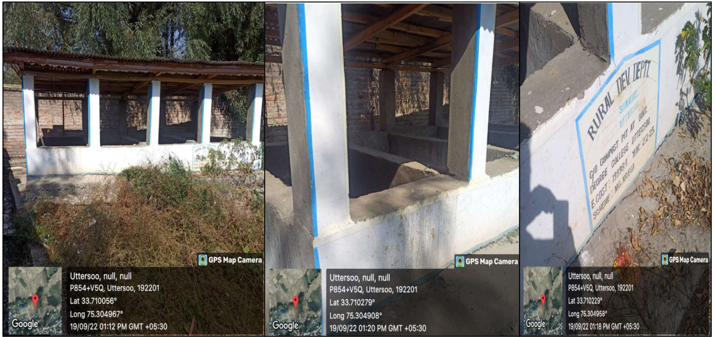
Waste segregation and composting facility
