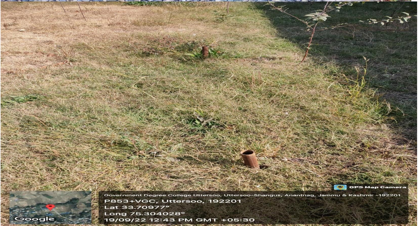
Rain Water Harvesting Structure
