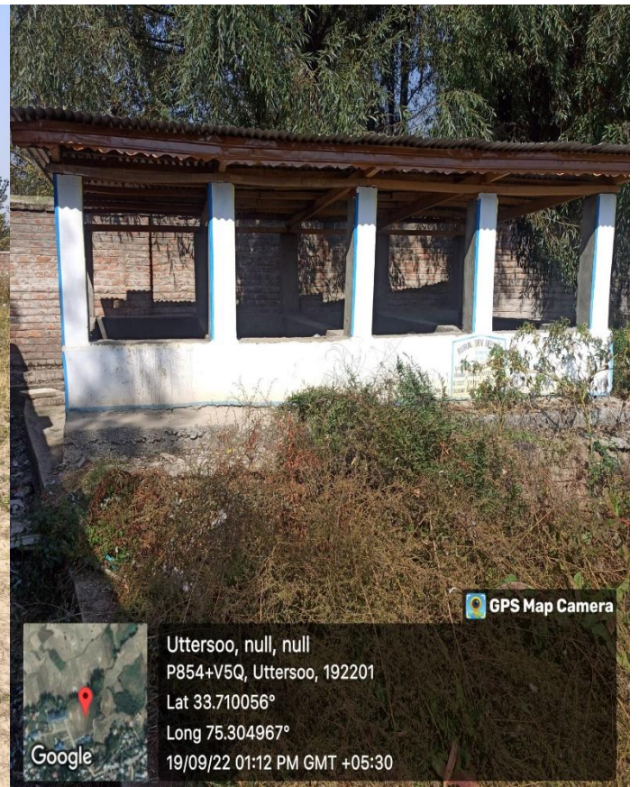
Waste Segregation Cum Compost Facility
