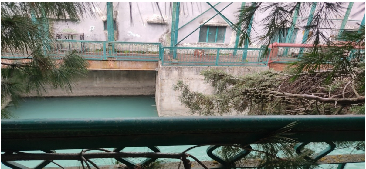
Hydro-Power project, Pahalgam
