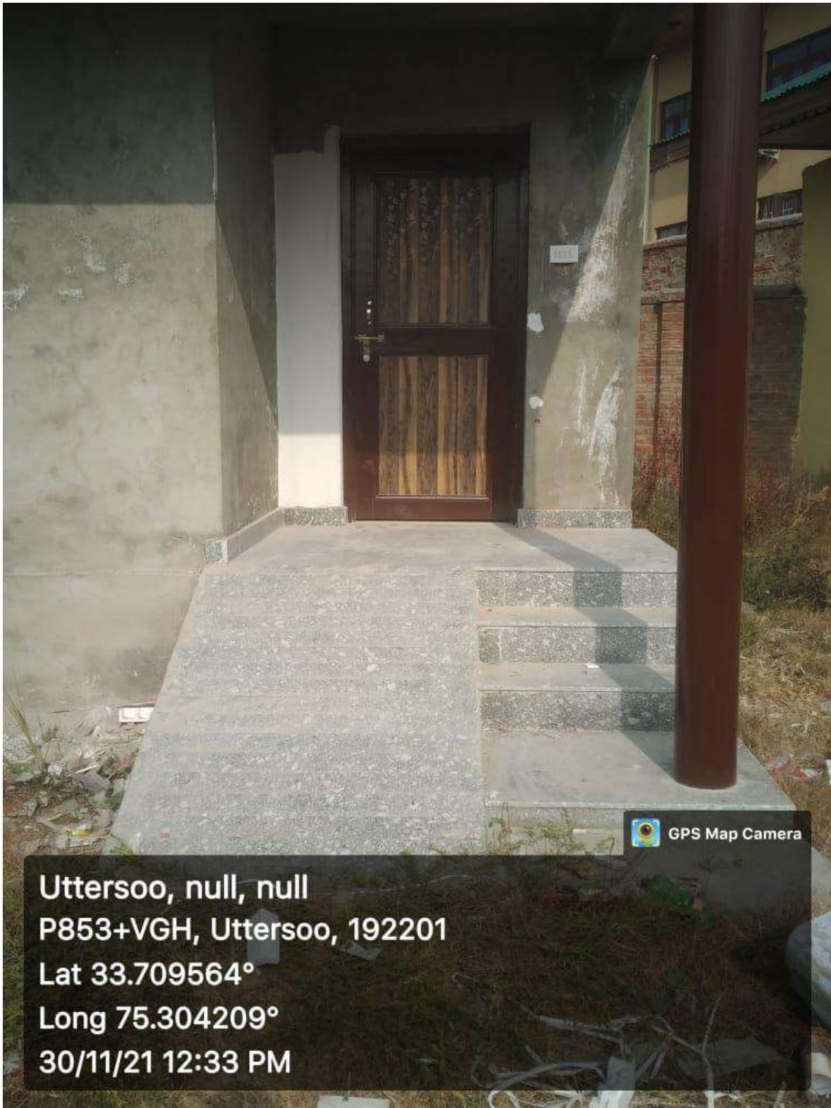
Figure 5 Ramp for Toilet Block (girls)
