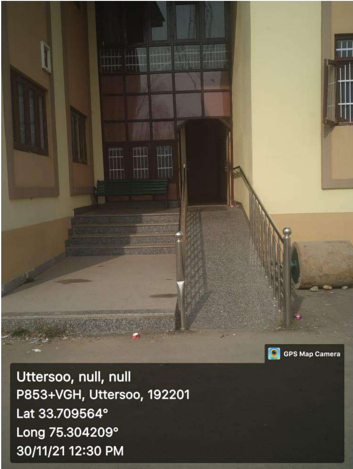
Figure 4 Ramp in the main building
